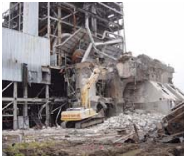
This project includes demolition and remediation of more than 30 facilities, including three generating units. The largest generating unit was imploded on January 13, 2007.
